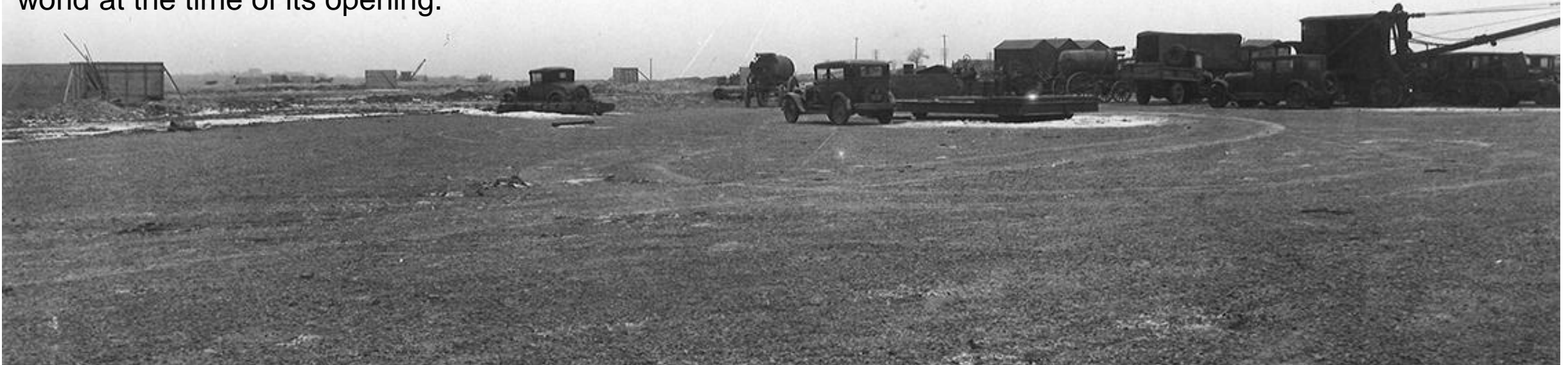
Photo: Construction site for new airport, December 1930
